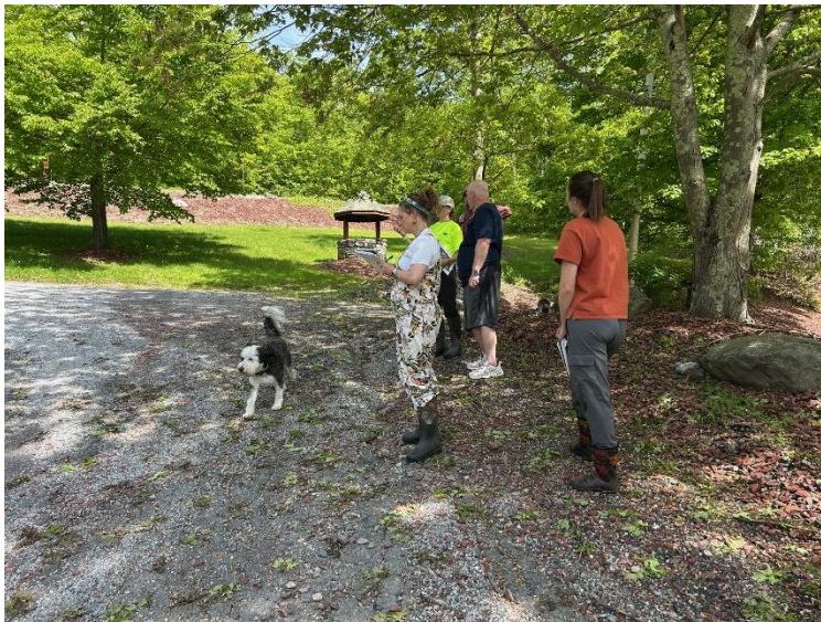
Photo 2: LL-01B – includes diverting runoff so it doesn't flow to this eroded section of gravel driveway (where PMNRCD and FEA staff are standing with a homeowner) but instead flows through a grassy conveyance to a bioretention basin (to the left of the photo).
