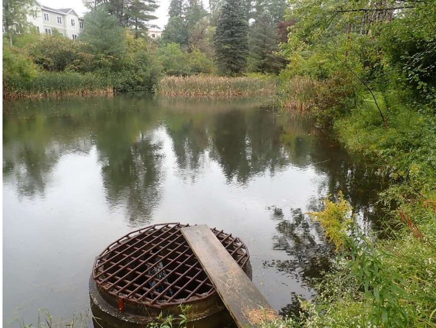
Campus Stormwater Pond Outlet Structure
