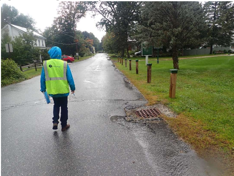
Catch basin on Seminary Street Functioning
