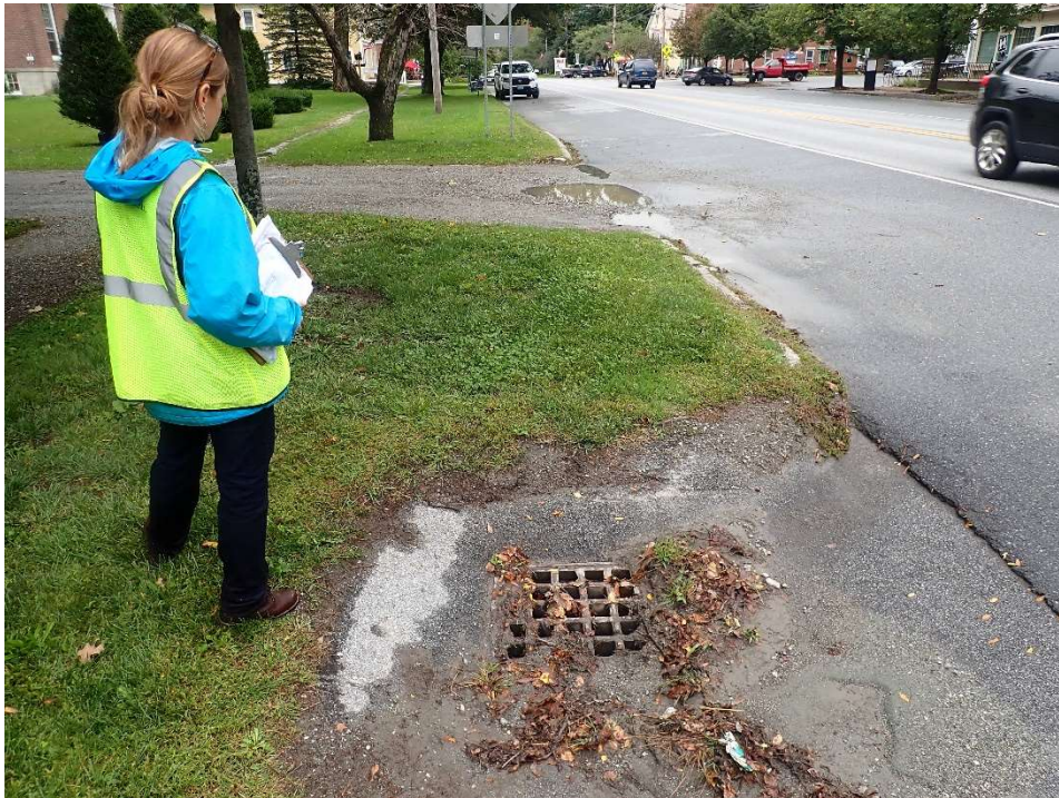
Material deposited at drop inlet near library driveway
