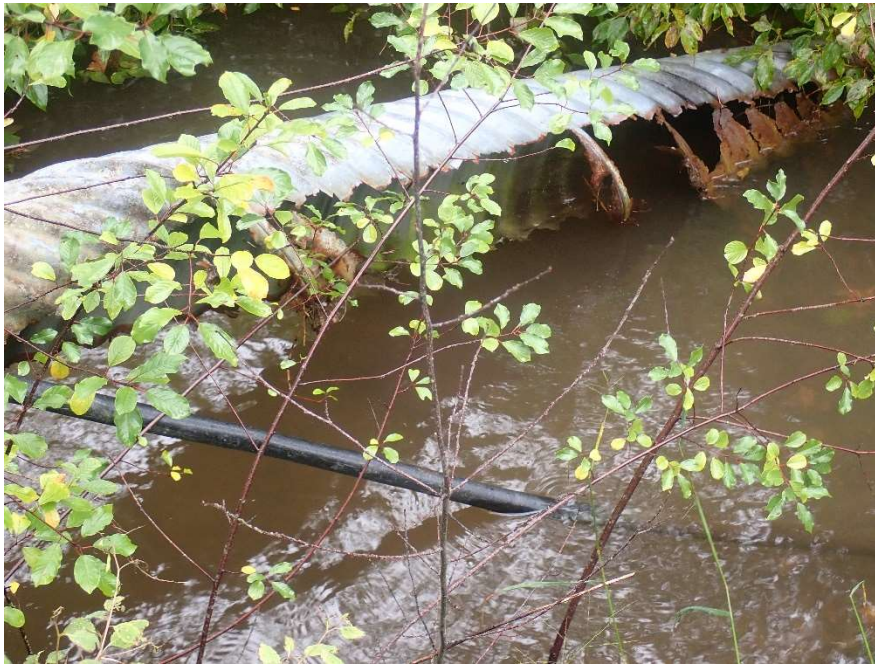
Pond Outlet Pipe Failed
