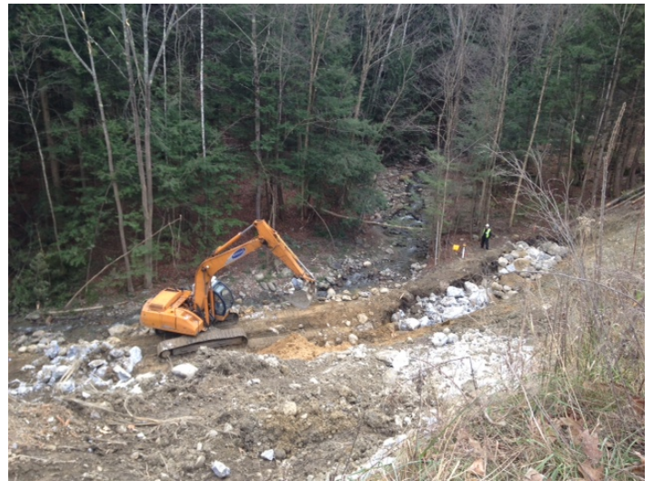
Dewey Avenue Slope Failure Restoration
