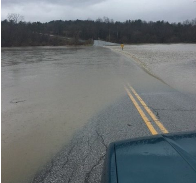
Inundation Flooding on Book Road
