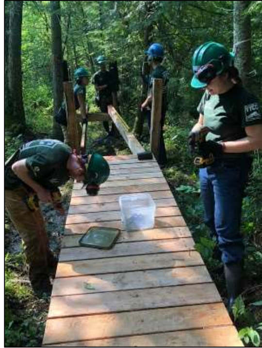
Figure 13: Marsh Trail Construction – Town of West Rutland
