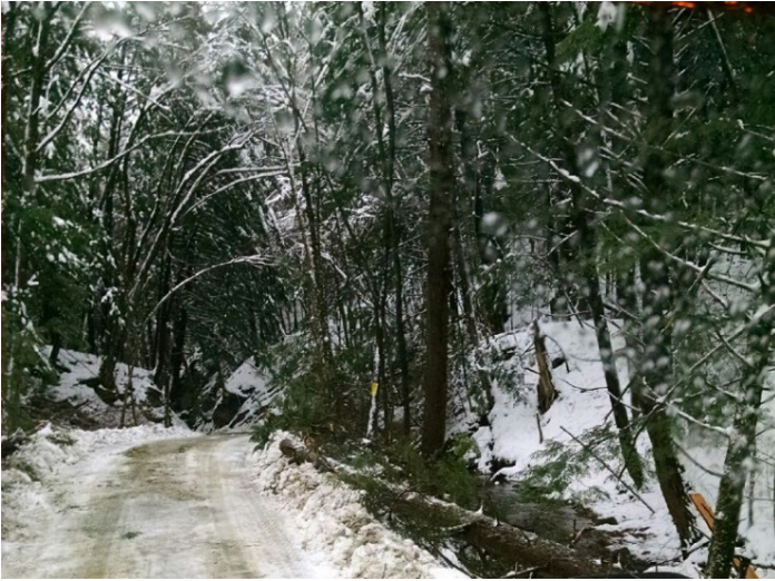
Dugway Road – December 2014 (DR4207) Storm Damage
