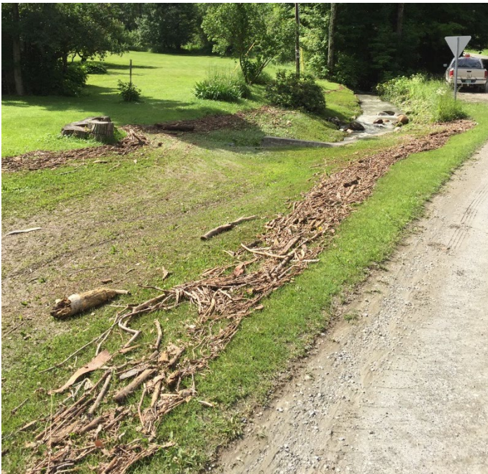
Debris from Flash Flooding at Gulf / Upper Gulf Road Intersection
