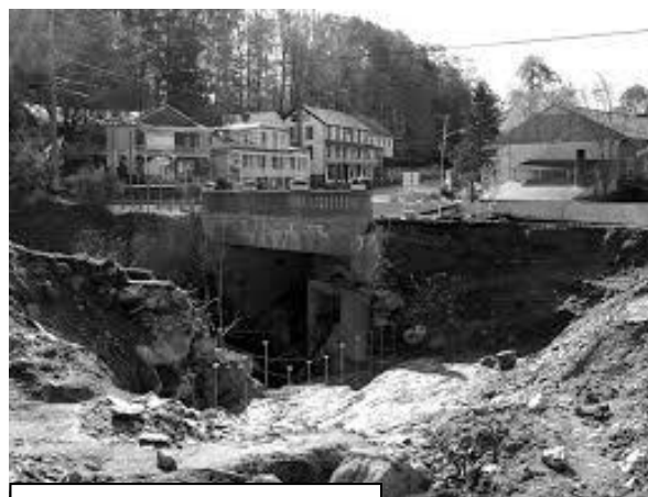
View of Route 30 Bridge from Cemetery Hill Road
