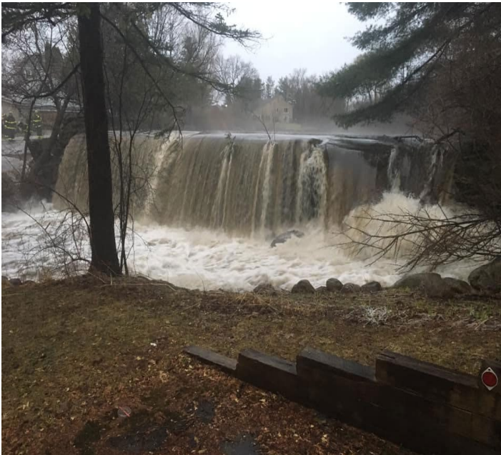
Dunklee Pond Dam overtopping in April 2019 (DR4445) – this dam was removed in 2021
