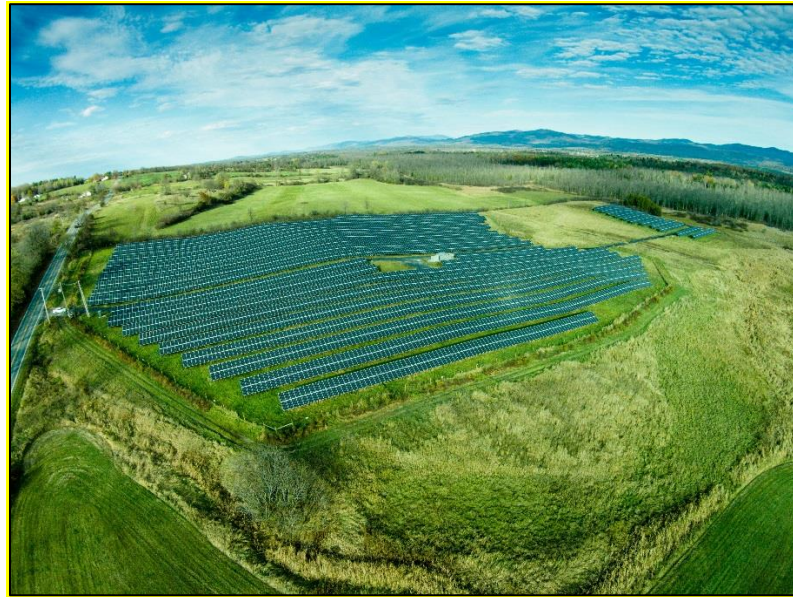
Sudbury solar project (2 MW) off Rt. 30 (courtesy Allco)
