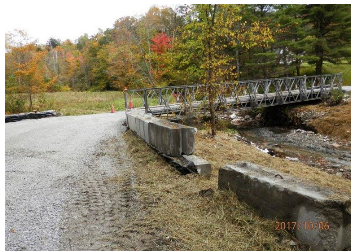
Parker Road Temporary Bridge - 2017
