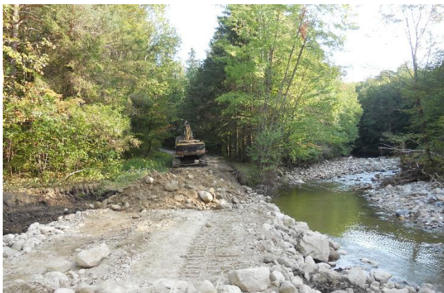
Casella Construction rebuilding Wheelerville Road after Tropical Storm Irene.
