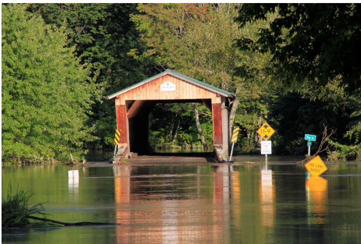
Gorham Bridge Flooding – Tropical Storm Irene 2011
