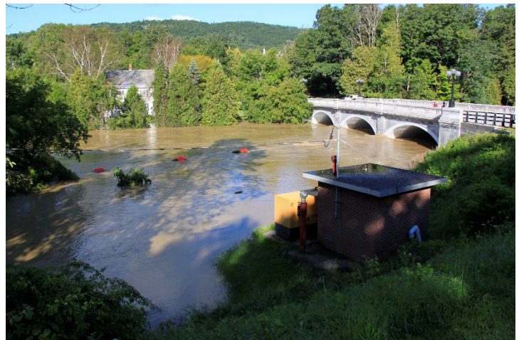
Otter Creek Floodwaters at Library Pump Station – Tropical Storm Irene 2011
