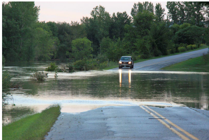
West Proctor Road Flooding – Tropical Storm Irene 2011
