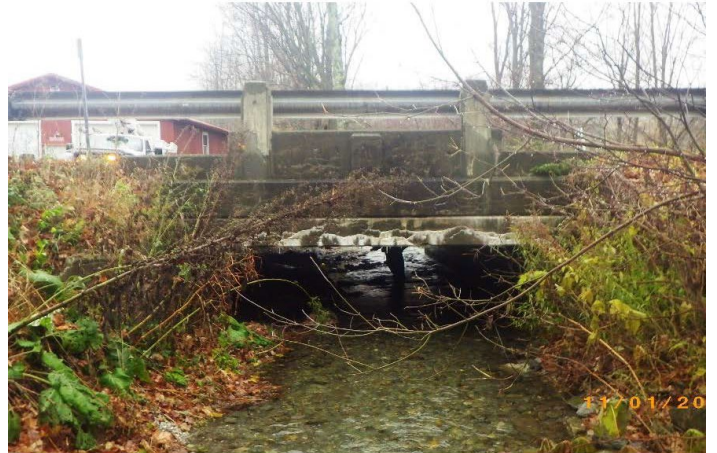
VT Route 133 State Bridge (B12) – 2018 (Ira Fire Station shown in background)
