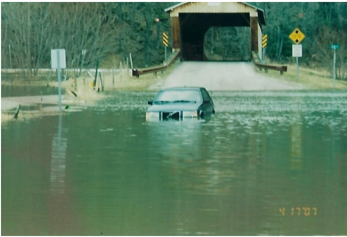
Inundation Flooding on Gorham Bridge Road
