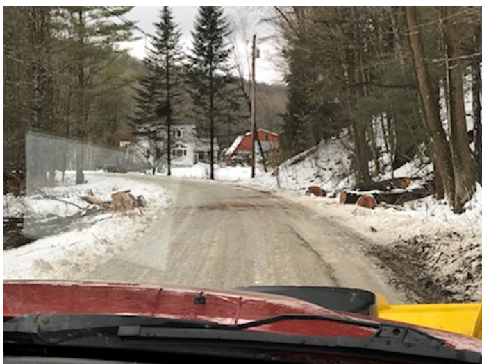
Ice Storm Damage – December 2018
