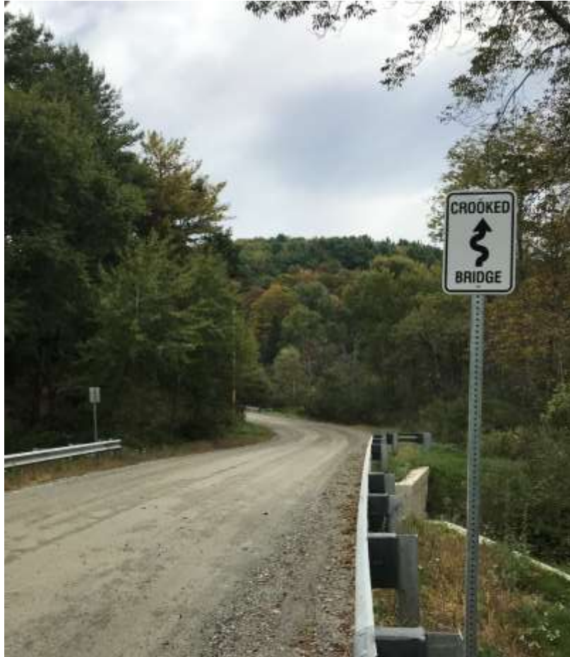
Fully Compliant Road Segment on Garron Road (RSID #101298)
