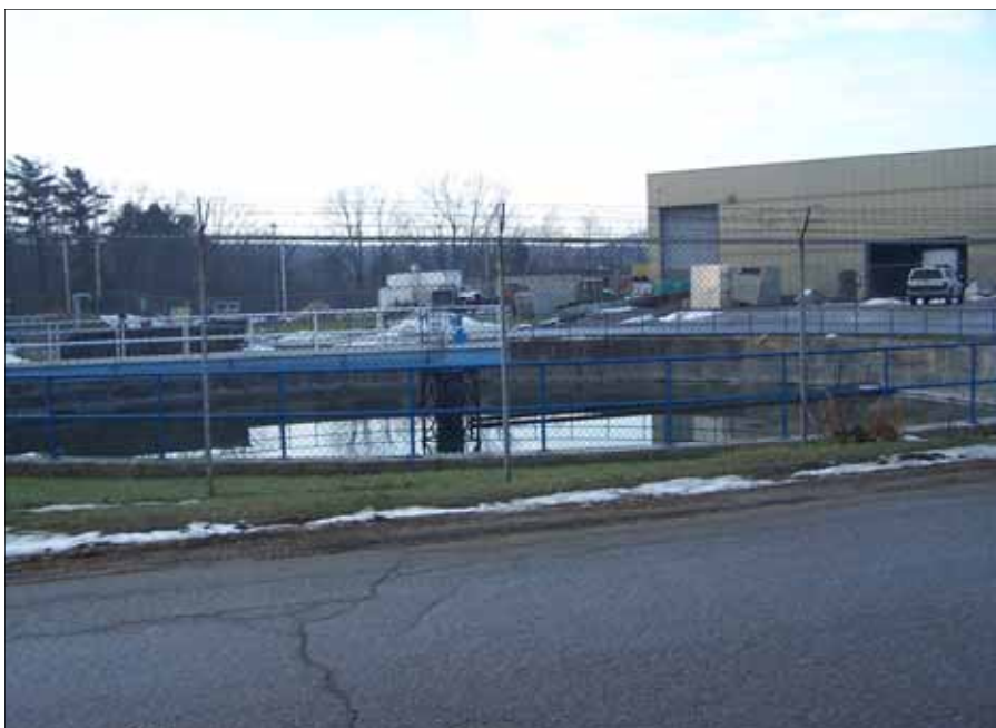
Wastewater Treatment Facility for the City of Rutland
