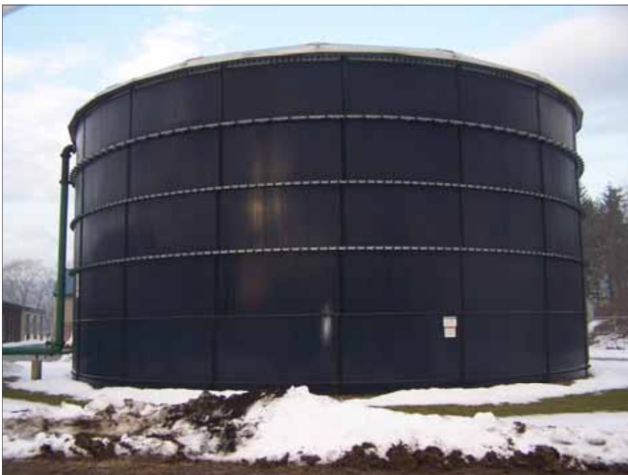
A municipal water supply serves the Village of Poultney.
