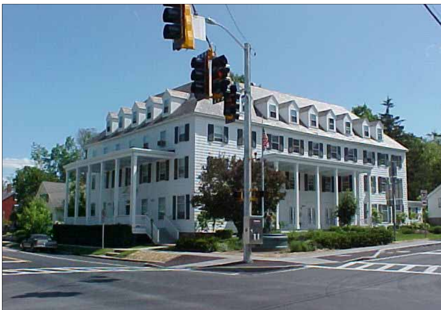
The Wallingford Inn provides subsidized senior housing in a historic village structure
